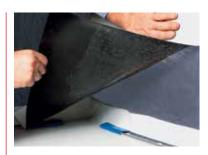
Bond the membrane to the upstand starting at the top edge and working down to the base.
