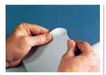
Heat and stretch the internal corner of the patch.
