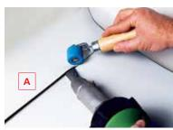
Spot-weld, pre-weld and weld the overlap on only the lower edge (A) of the horizontal surface.
