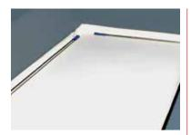
It is always necessary to fix around the perimeter with a pre-drilled TEXSA bar. The bar can be mechanically fixed on the horizontal or vertical surface at the base of the upstand.
