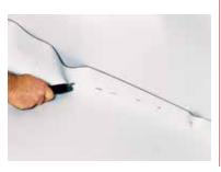
Install the TEXSALON field sheet. Bond and cut the membrane to form a bend of approximately 3 – 4 cm on the vertical wall. Once in position, cut the excess material to create a minimum upstand of 2 cm.
