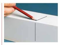
Squeeze the drip near the cutting line to identify the desired cutting point.
