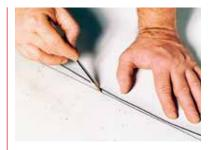
Bend back the new material. Clean the surface of the existing membrane with an abrasive disk.
