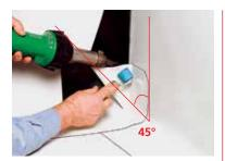
Spot weld in position as indicated. Then fold the membrane to form an upright crease.
