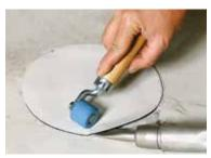
Spot-weld, pre-weld and weld the patch in place.
