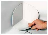
After chamfering the seam edge, spot weld the TEXSA TPO prefab corner in position.
