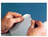
Round the corners of a square patch of TEXSALON TPO unreinforced membrane (TEXSALON SA) allowing a 2 cm excess for overlapping and welding. Heat and stretch the internal corner of the patch.
