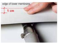
1.4 Phase 1 – spot welding Spot-weld the overlap, about every 40 cm. Distance the spot welding from the edge of the lower sheet, by:
