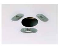
Mechanically fix the membrane around the outlet to the decking withy fixing plates and screws.
