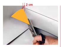
Overlap the two edges of membrane and cut the excess material up to 2 cm from the edge as illustrated in the picture.
