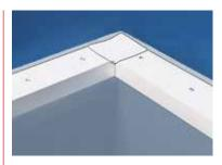
Spot-weld the flashing onto the profile starting 1 cm from the edge. The excess membrane from the vertical surface will form a pocket at the corner edge.
