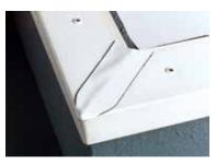
After positioning the neoprene or butyl sealing strip, mechanically fix the prepared flashing to the perimeter edge. Cut and weld a strip of
