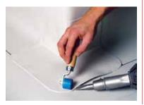
Spot-weld, pre-weld and weld working from the centre of the corner outwards.
