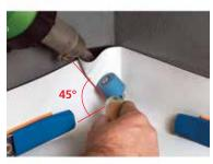
Fold the excess membrane towards the wall.
