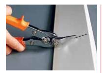
Cut the horizontal surface following the cutting line.
