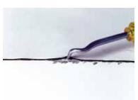
In the case of defective seams, follow the seam cleaning procedure prior to re-welding as necessary. In extreme situations, it is necessary to weld a 15 – 20 cm strip over the existing welding line after cleaning. When using automatic welding machines for this process use the TEXSA SCRAPER NOZZLE. (see point 15).
