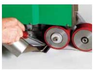
b) automatic welding with Varimat welder Position the new TEXSALON TPO on the existing membrane. Mark the overlap line. Bend back the new material.
