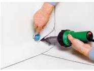
Close the bend on the vertical wall by spot-welding, pre-welding and welding.
