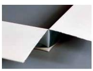
Open the flashing. After installing the neoprene/butyl sealing strip, mechanically fix the flashing to the perimeter edge.
