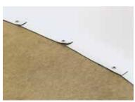
Cut the membrane and weld the excess material as indicated.
